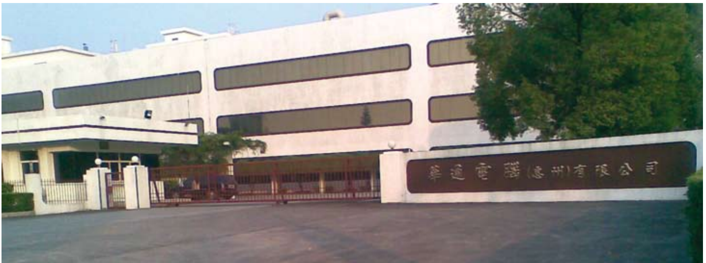
Compeq Factory in Huizhou, Guangdong. Source: SACOM.
