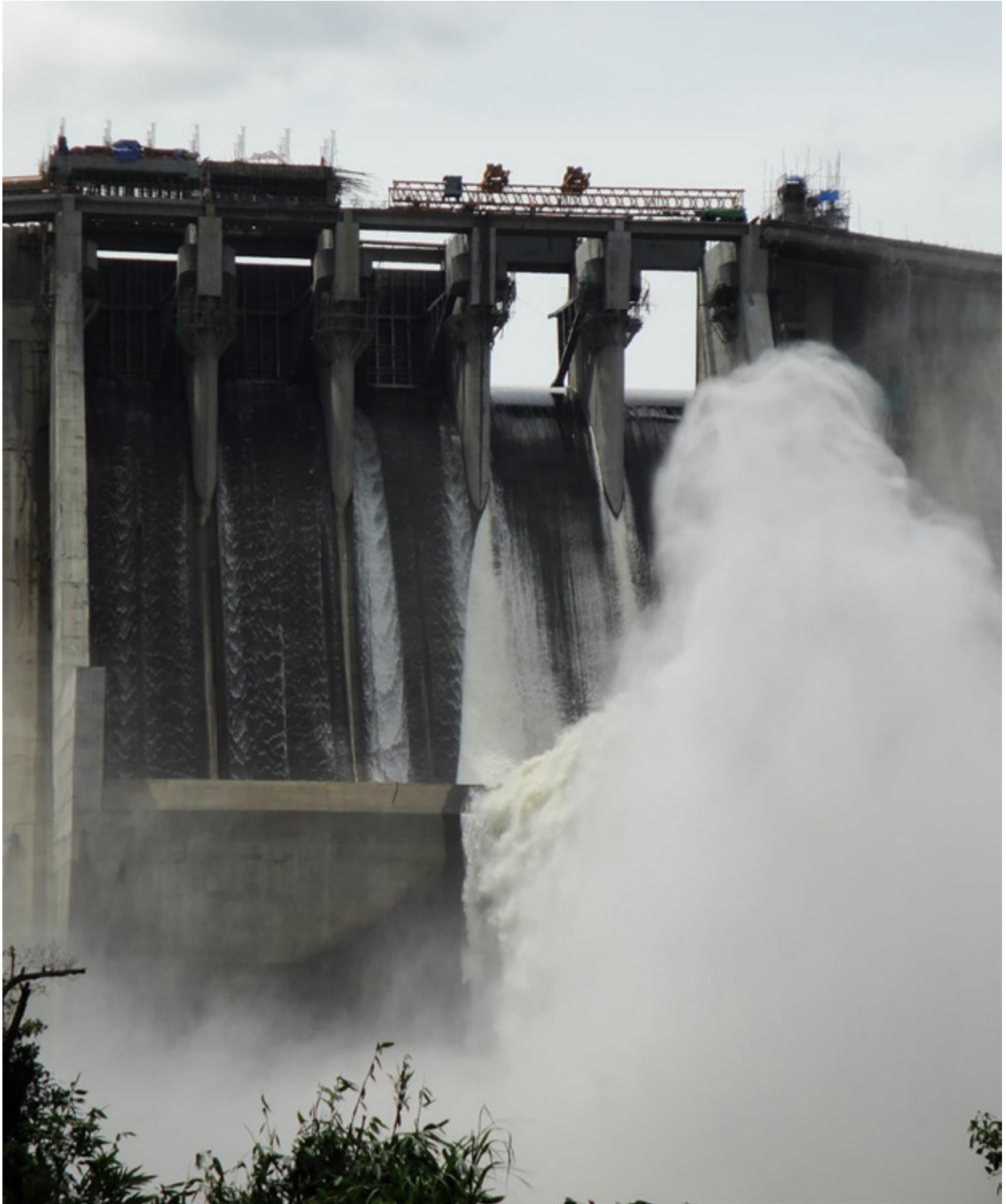
Kamchay hydropower dam, Cambodia, operated by Powerchina Resources (by Inclusive Development International)
